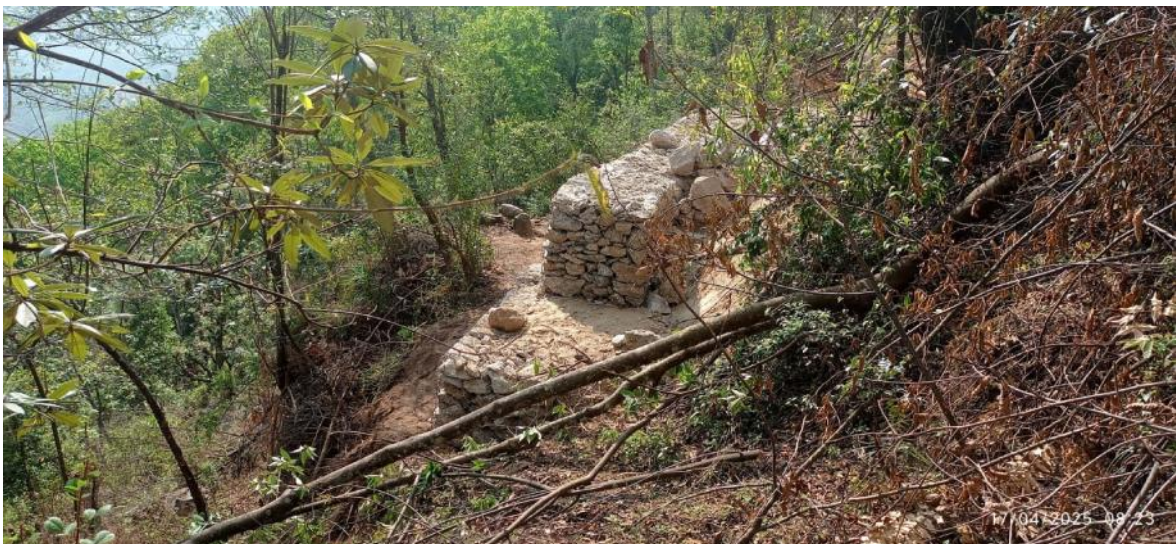
Fig. Ongoing construction of gabion wall for slope stabilization and protection along the access road of Pegu Khola Small Hydropower Project.
